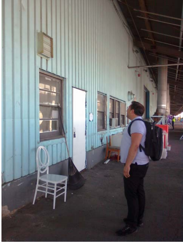
Current exterior, seen from loading dock
