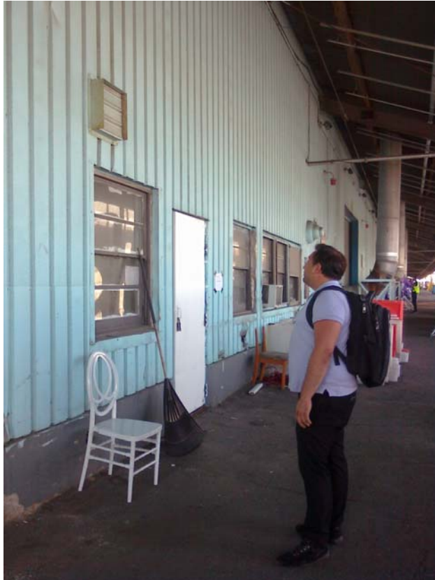
Current exterior, seen from loading dock
